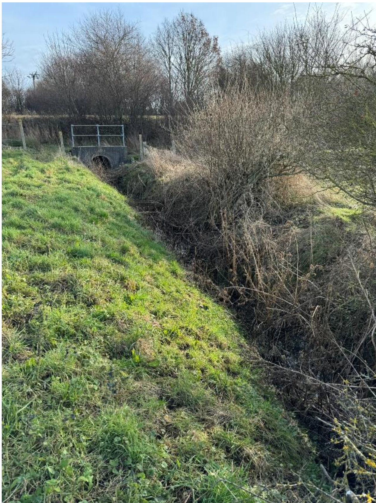
Photo 11 – Central Ditch/ A10 Culvert
