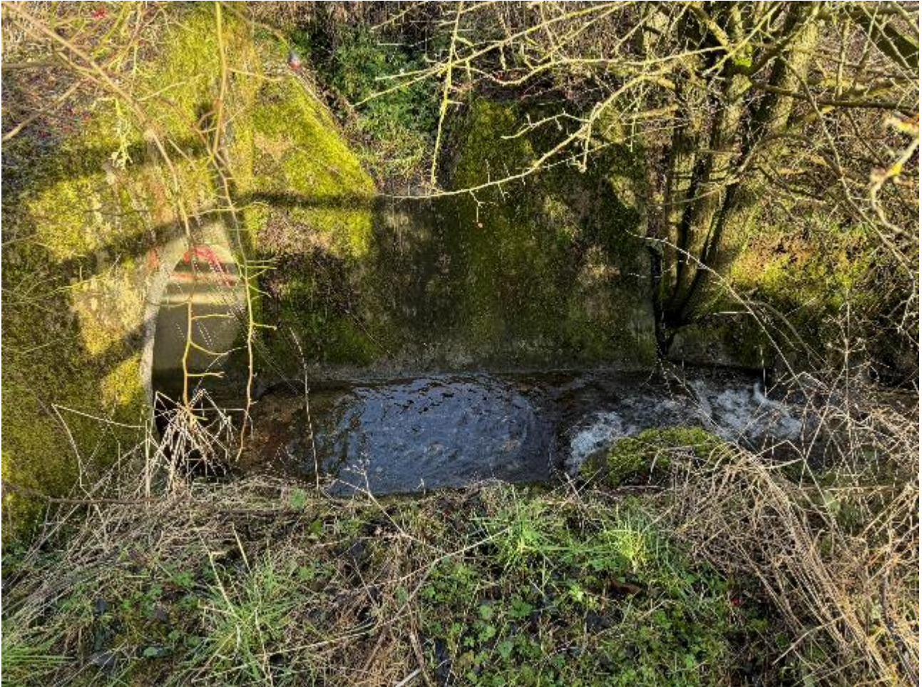
Photo 7 – A10 Culvert/ Ordinary Watercourse to East of A10
