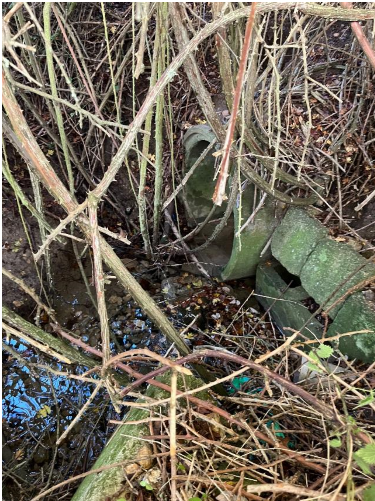
Photo 4 – Existing North-East Drainage Ditch Culvert
