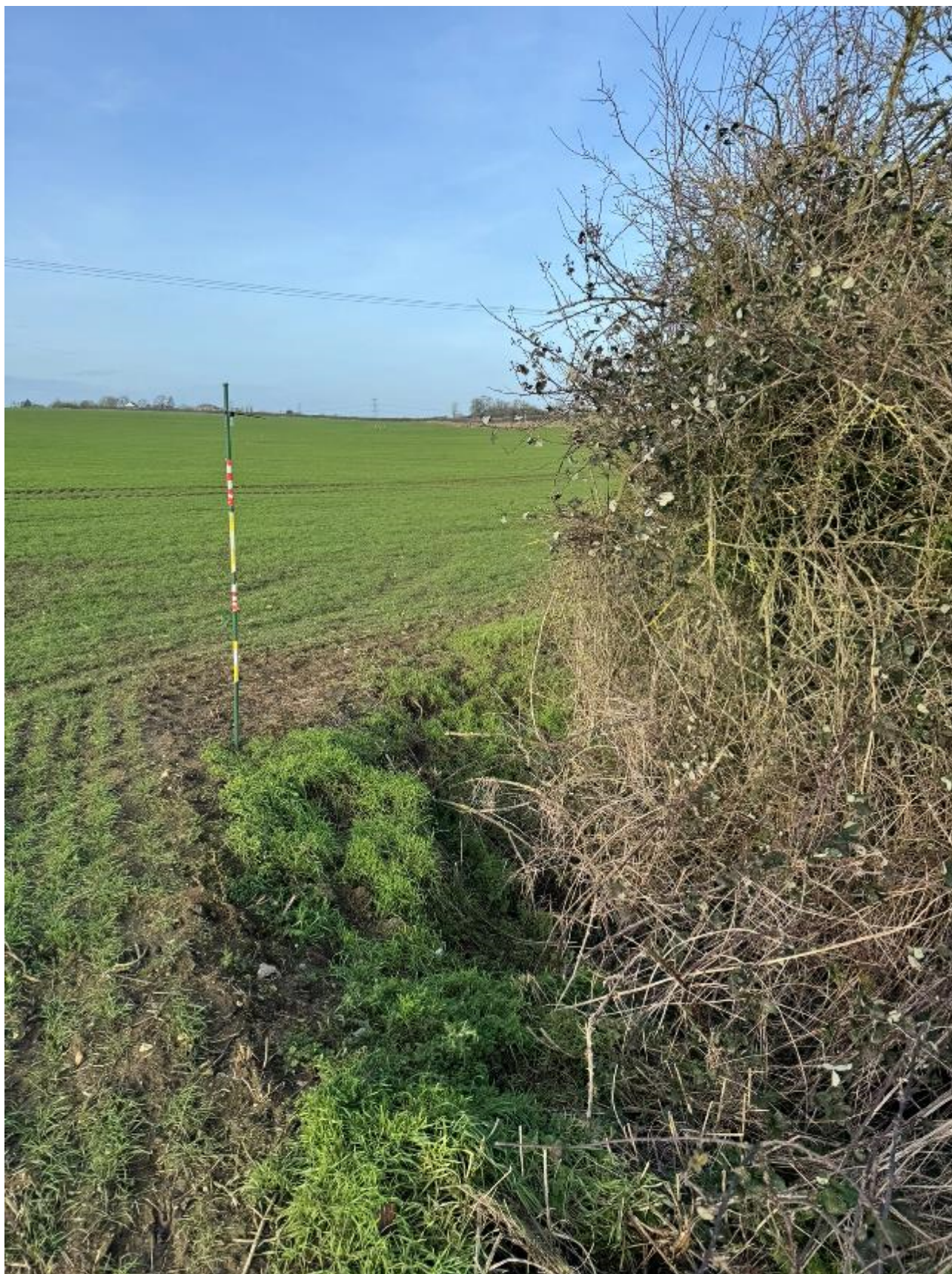
Photo 3 – Existing North-East Drainage Ditch at Site Low Point
