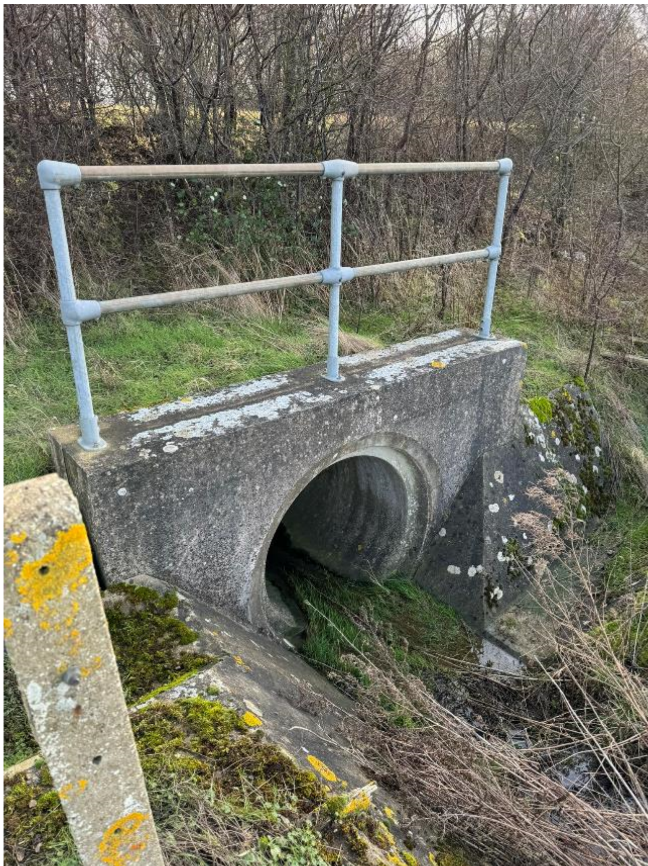
Photo 13 – Central Ditch A10 Culvert
