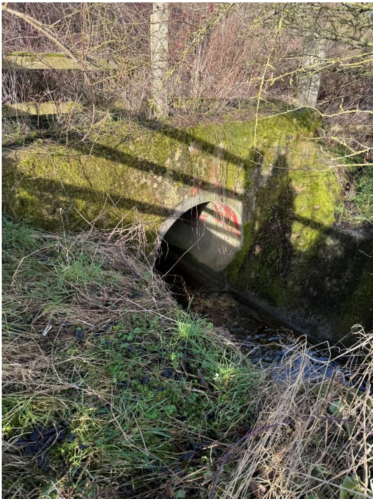
Photo 6 – Culvert Beneath A10
