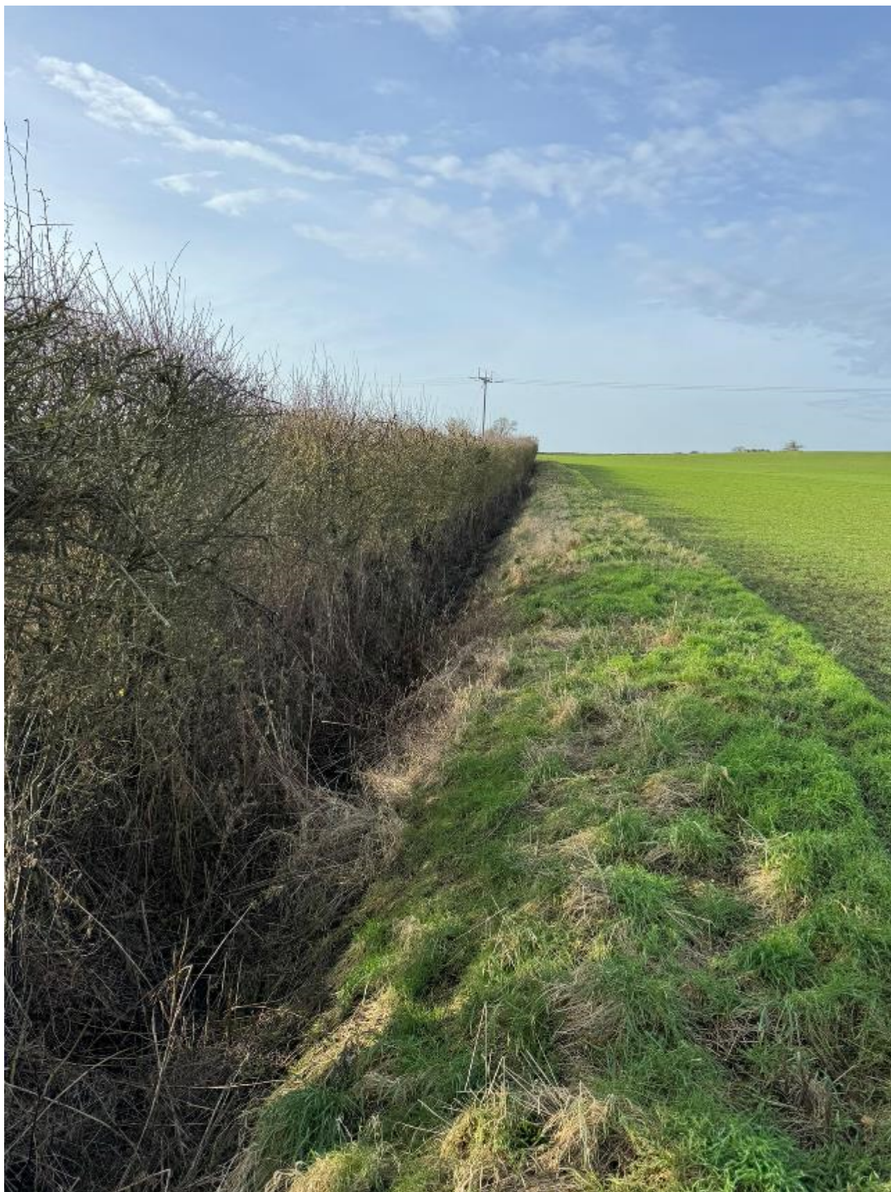
Photo 10 – Central Drainage Ditch
