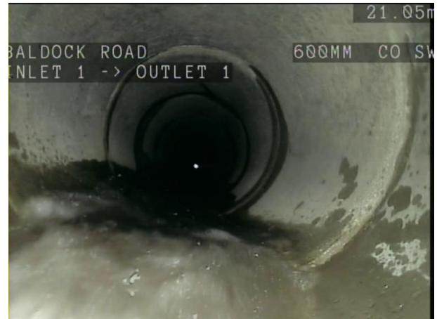
INLET 1X_2d35a7fd-a5d7-4f11-b3eb-28676845b3c7_20241209_102 451_929.jpg, 00:02:29, 21.05 m General photograph taken at this point, 2.25
