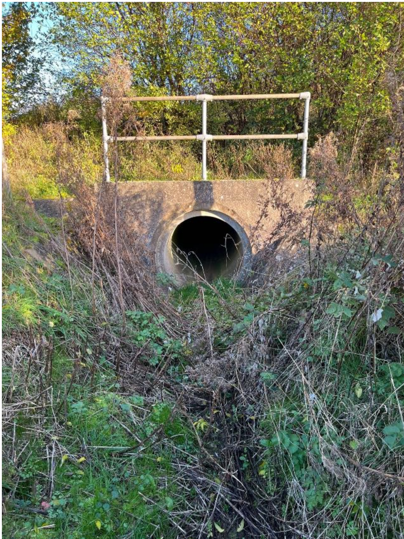
Photo 12 – Central Ditch A10 Culvert
